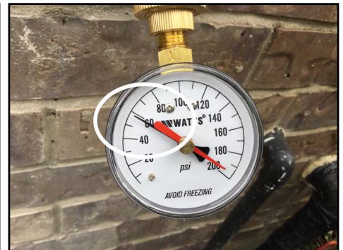
PSI measured between 56 - 60 range during inspection
