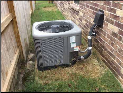
Right exterior condenser unit inspected
