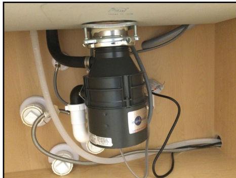
Kitchen sink disposer unit inspected
