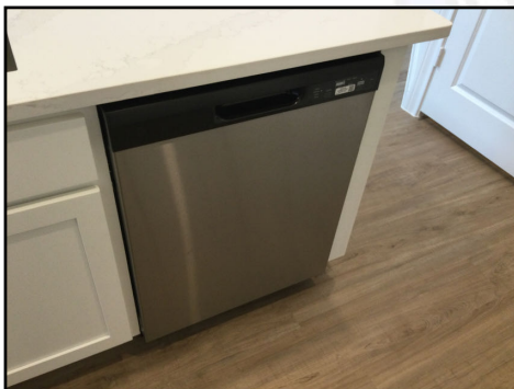
Kitchen dishwasher unit inspected
