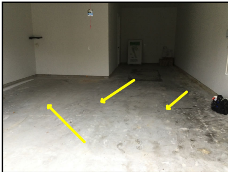
Interior garage surface cracking observed across flooring locations (Cracking did not appear to have any bearing upon foundation performance during this inspection. Recommend monitoring for future performance)
