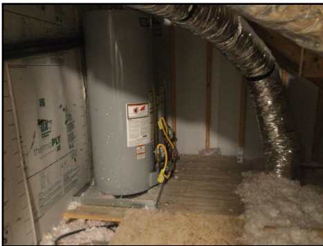
Attic water heater units inspected
