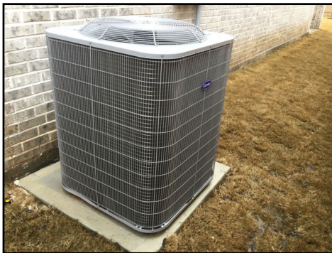
Right exterior condenser unit inspected
