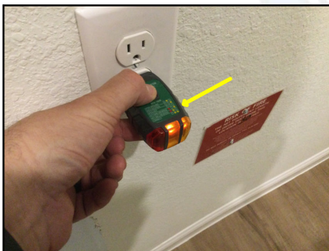
Utility room receptacle not GFCI protected (Recommend an electrical contractor for further evaluation)
