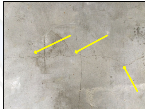
Interior garage cracking observed across flooring surface.
