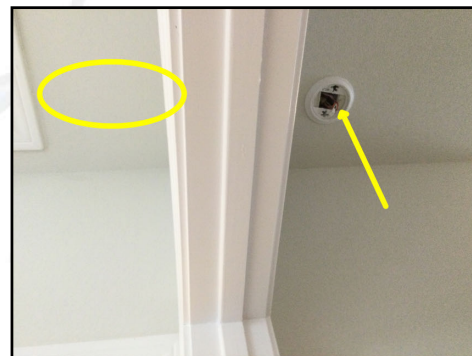
Smoke/carbon monoxide detector not present at back upstairs bedroom
