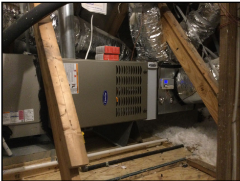
Attic furnace unit inspected
