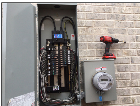
Right exterior distribution/disconnect panel inspected
