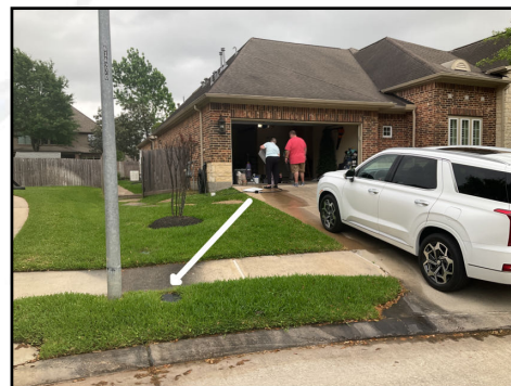
Water meter located along front left exterior
