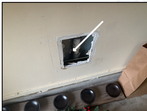
Water shutoff appears to be located along left interior wall
