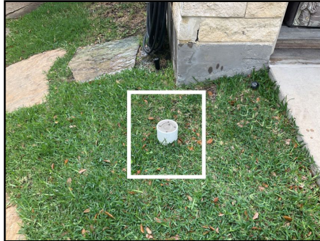
Sewer tap observed along front exterior
